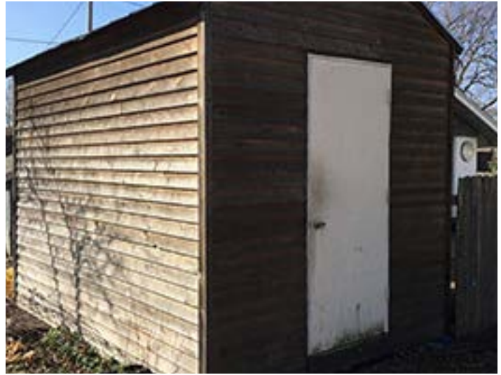
Jessi Asmussen and Kevin Prather built a two-zone walk-in refrigerator at their home. The unit is built on pallets and can be moved by forklift.
